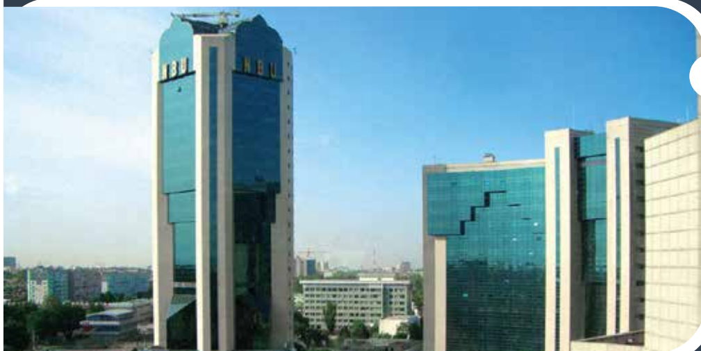
NATIONAL BANK OF UZBEKISTAN COOLING SYSTEM REVISION - 2021-2022
