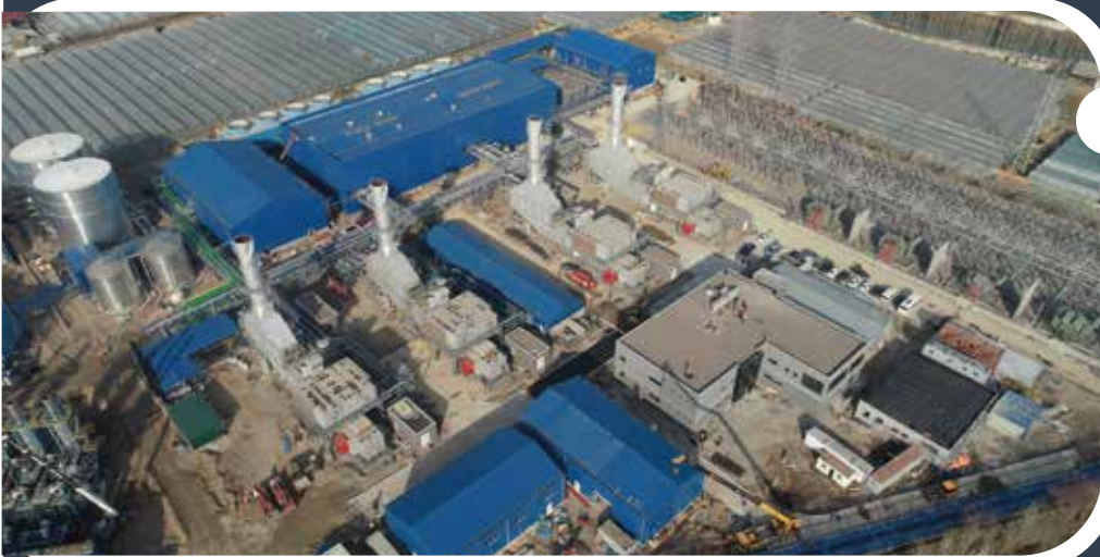
AKSA ENERGY PLANT A CCPP 240MW – 2022
