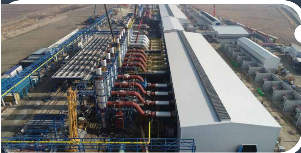
AKSA ENERGY PLANT C CCPP 270MW – 2022
